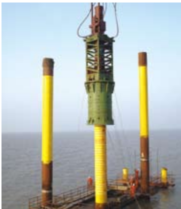
天津渤海湾石油平台D220柴油锤 Bohai Bay Offshore platform, Tianjing. With D220
