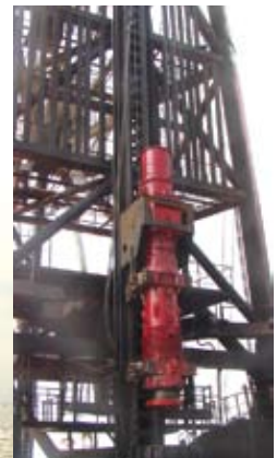
东海风电一期二期D220柴油锤 Donghai Bridge Wind farm, Shanghai. With D220
