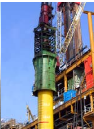
天津渤海湾石油平台D220柴油锤 Bohai Bay Offshore platform, Tianjing. With D220
